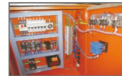
24V LVDC power for control system, more secure and reliable
